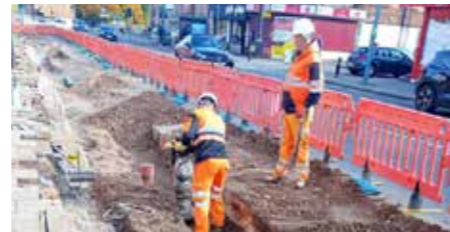
Working at Dudley Road in Birmingham
