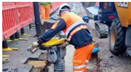
Yorks Bridge in Walsall
