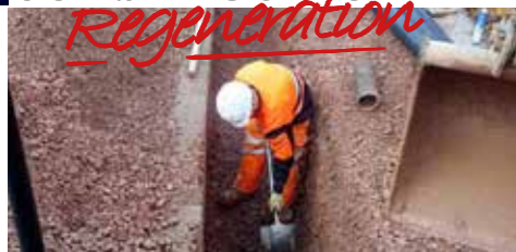
The groundworks training area at Telford College
