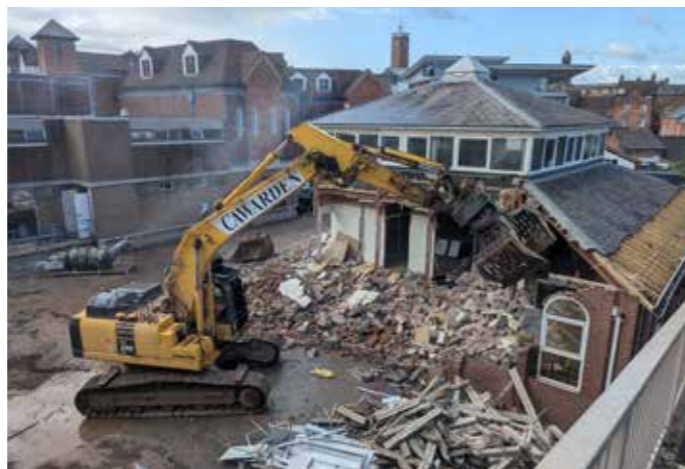
Demolition of the Riverside Centre has begun
